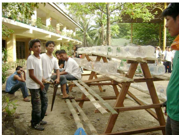
Students constructing the container garden structure
