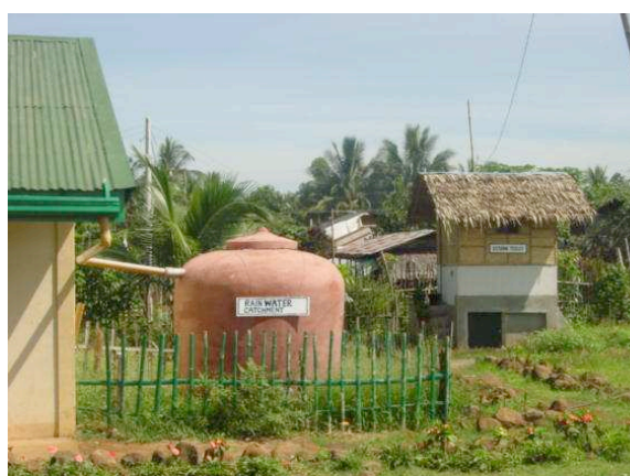
A rainwater catchment in Balubal National High School with the Ecosan toilet in the background
